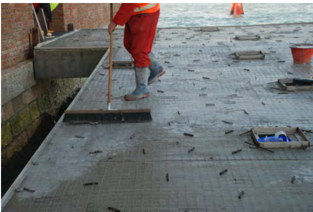
1. Application of adhesion promoter, Bonding Agent and cement slurry.
