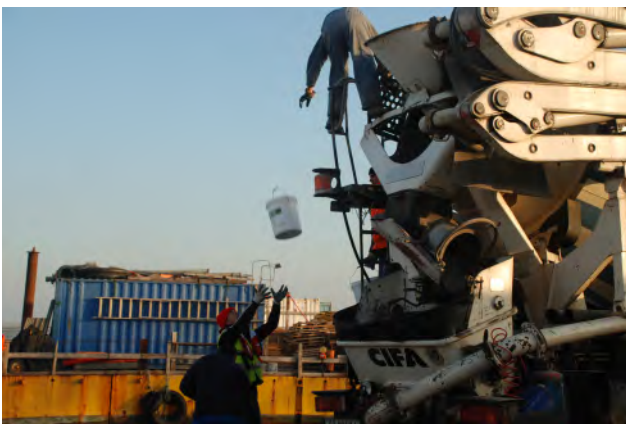
2. Adding Bonding Agent to the concrete directly in the mixer.
