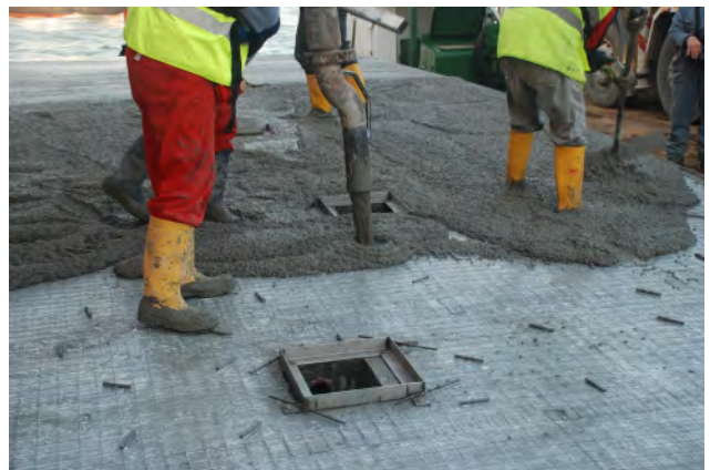
3. Laying the concrete. In this case, it was possible to create a new 4 cm thick pavement.
