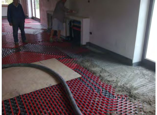
Low-thickness screed above underfloor heating
